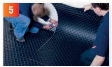
Once primer has dried start by laying the egg crate panels onto the floor peeling off the plastic sheet as you go so that they stick firmly to the floor. Please ensure that the panels overlap one another on the appropriate sides. You will notice on the panel, two of the sides have smaller nodules, these are designed to go underneath the next adjacent panels and push together.
