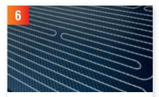
Once the panels have been laid, install the underfloor heating pipework, 12mm pipe at 150mm centres (unless designed differently), and connect to the manifold.
