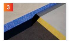
Ensure the floor is clean and dust free, then fix the foam edging insulation around the perimeter and seal any holes that may allow levelling compound to leak into.
