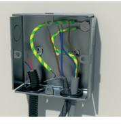
The earth from the mat can then be connected to the earth from the incoming supply by using the earth terminal in the back box. If using a plastic box with no terminal then a terminal block can be used.
