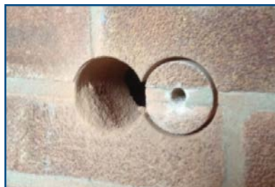
2. Drill two 65mm holes next to each other.
