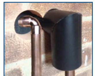
4. Fit the elbow over the copper pipes
