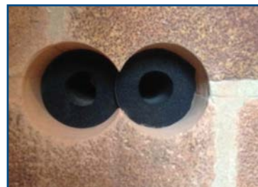
3. Insert the PVC sleeve insulation, recess it to allow for the elbow to be located.
