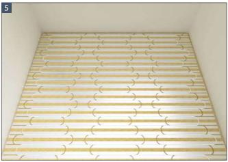
• Following the projects working drawings, begin laying the pipe, pressing the pipe into the channels.
