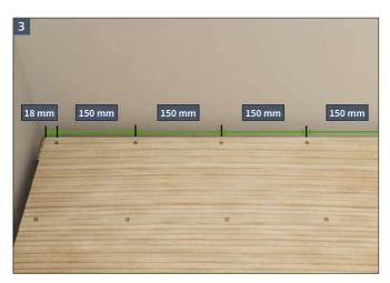
• Screw the plywood covering into the Econna-12 panels using 25 mm wood screws, 18 mm in from the edge of each plywood sheet and then at 150 x 150 mm centres, ideally in the centre line between the pipe runs.
