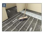
Before installing the pipework ensure the adhesive has cured where used. Sweep or vacuum the panels to clear any debris.
