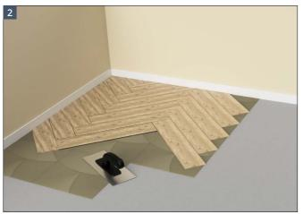
Lay the floor covering adhering to the flooring manufacturers instructions. If gluing the floor finish ensure the adhesive is suitable for use with underfloor heating.
