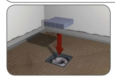
13. Place the Disposable Tiling Aid into the shower drain hole on the Shower Tray. The Tiling Aid provides the edge that needs to be tiled up to whilst protecting the Shower Drain from debris.
