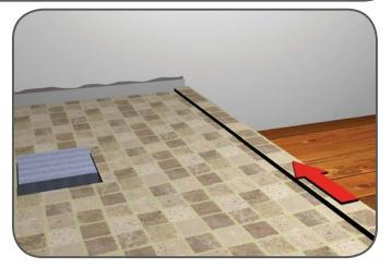
14. (Optional) After tiling the base of the shower area, we recommend that you add a further narrow border of tiles approximately 30mm to 40mm wide, along the top of the outside edge to act as a water retainer, stopping water running out of the shower area. The tiling aid can now be removed and disposed of.
