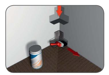
9. **Note:** Wear protective gloves, eye and breathing protection. Apply a thin layer of Pro-SEAL tape sealer to the internal corners of the shower area, slightly bigger than the pencil line marked in step 8.
