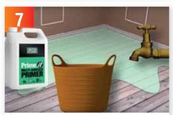
Whilst the primer on the boards is drying commence with priming of the substrate using UltraFloor Prime-IT MSP. The primer should be diluted 3 parts water to 1 part primer and allowed to fully dry.
