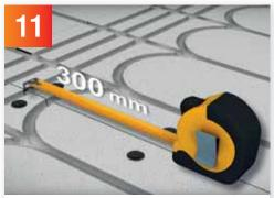
Additional use of ProWarm™ screws and washers is recommended over timber substrates where needed, fixed at every 300mm.
