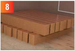
Allow the floorboards to acclimatise to the indoor room temperature for at least 24 hours as they may swell or shrink depending on the climate.
