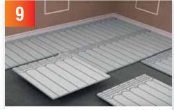
Bed the boards, primed side down, into the adhesive and ensure compression of adhesive ridges, ensure full compression of the adhesive to give a void free full adhesive bed.
