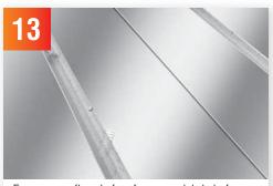
Ensure your floor is free from any debris before installing the pipe. It is important to check in all the grooves as the pipes could be damaged during installation if there are any obstructions.
