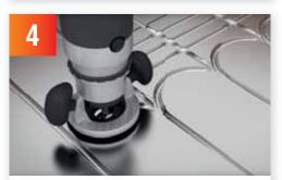
You may be required to modify the heating panel to navigate around permanent fixtures. If you find you need to create a new channel then this can be done with a knife or router.
