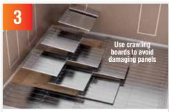
Loose lay the boards across the floor and number the boards on the upper face to identify position of each board, making sure the pipework runs are calculated correctly to reach manifold position.
