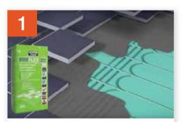
Fix the tiles using UltraTile ProFlex S2 adhesive. Ensure that every pipe channel and void surrounding the pipe is fully encapsulated with tile adhesive.
