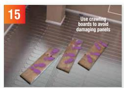
Try and limit the amount of walking on the boards, and where possible lay boards to prevent indentations on the boards.
