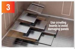
Lay the boards across the floor with the grooves facing upwards, making sure the pipework runs are calculated correctly to reach manifold position.
