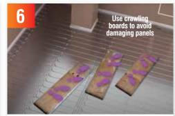
When laying the boards it will be inevitable to need to walk across them, but try to keep this to a minimum level where possible.
