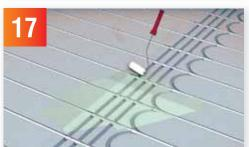
Prime the upper face of the boards with a neat coating of Ultra Prime-IT MSP bonding primer. This should be applied by brush or roller in a thin film. Allow to thoroughly dry to a clear green film, (approx 1-4 hours).
