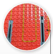
The cold tail joint can be secured in place by taping the cable either side of the joint, a small piece on the heating cable and a small piece on the cold tail. This will ensure the joint is NOT covered with tape.
