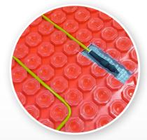
The end joint can be secured in place by taping the yellow heating element just before the joint to help secure it in place. This will ensure the joint is NOT covered with tape. Both these heating joints MUST now be fully encapsulated within levelling compound and/or tile adhesive.
