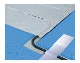
When installing two or more ProWarm™ heating mats next to each other make sure that the heating wires in adjacent mats DO NOT overlap. We recommend the use of adhesive tape to ensure that they will not move over a period of time.
