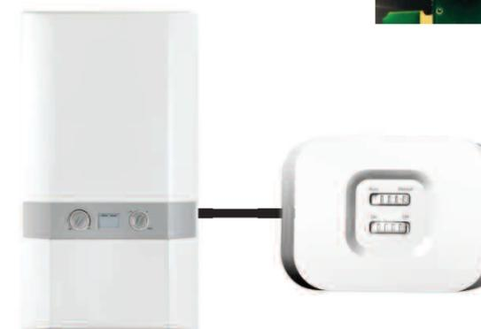
System Receiver configured to boiler receiver RX1. Refer to reverse side for wiring.
