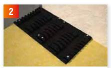
Start by laying the first two End Supports into the corner of the room and fix to the wood floor using the available screw holes. Alternatively, if fitting onto a concrete floor, then use either the Overlay adhesive to bond the returns to the floor. or fix directly through to the concrete by raw plug and screw.
