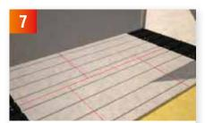
Upon completion of the first row. start the process again by placing two more Overlay End Supports next to the existing ones, and secure with the integral inter-locking points. Following this, you will need to work your way back up the room, staggering the panels as you go. Ensure you apply the 3mm bead of Overlay glue to all edges.
