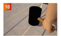
Start to push the pipe into the Overlay, ensuring the pipe is fixed beneath the surface of the board (preferably using a soft rubber mallet or your foot to ensure a good fixing)\*
