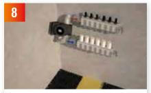
Start by fixing the 1515 manifold to the wall, about 500mm from the floor to the top of the flow meters. Connect the first circuit to the manifold with the euro cone adaptors.
