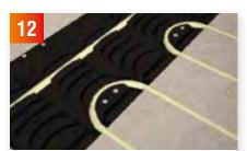
Continue to lay the pipe along the room until you reach the opposite end by walking the pipe into the groove as you go. Once you reach the end of the room, use the End Support to return the pipe back towards the other end.
