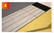
Upon approaching the end of the first row. place two Overlay End Supports into the corner up against the wall. This will leave a final cut of the Overlay to complete the first row. if required.
