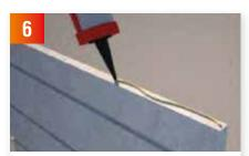
Work your way back up the room, staggering the panels as you go. Ensure you apply the 3mm bead of Overlay glue to all edges.
