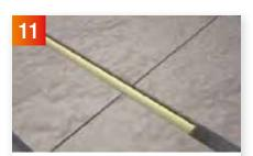
Use a small piece of the underfloor heating pipework to place in between the groove joining two boards. This will help to keep the floor in place.
