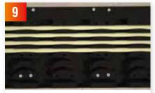
Start to roll the pipe into the Overlay End Support, utilis ing the selfretaining pipe clips, and continue to push the pipework into the connecting pipe runs until you reach the other end of the room. When rolling out pipe if possible please use a pipe de-coiler, if not available lay pipe flat on floor and feed out pipe sideways. Do not roll pipe like a wheel as this causes the pipe to come loose and not hold in place as well.
