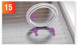
Above picture: illustration purposes only, ideally the pipe should be unrolled using a de-coiler or in the horizontal position to allow for ease of laying the pipe (This will stop the pipe trying to spring out of the boards at the end of the panels).
