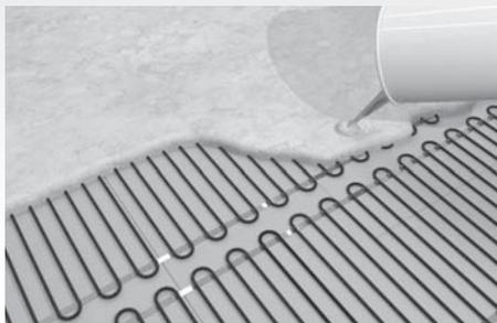
If you are using a suitable vinyl/ carpet or engineered/laminate floor as the final covering then we recommend a minimum of 8mm suitable latex levelling compound to cover the heating mat/cables to ensure even heat distribution.
