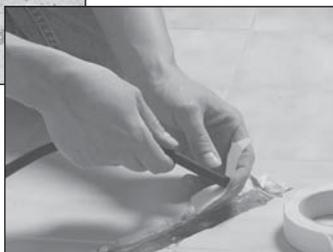
It is important that the channel is positioned such that it lays between two heating wires and not across them and not above heating pipes below the floor. The end of the tubing in the floor is sealed with tape to prevent adhesive entering the tube.
