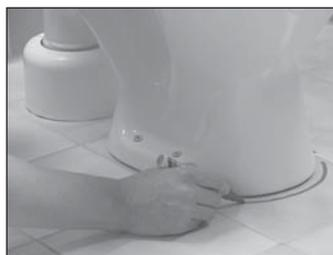
3. Each mat is supplied with a piece of 10mm flexible tubing (only one tube is required for each thermostat), this is for the floor sensor, so that in the unlikely event that the sensor fails, it can be easily removed and replaced without lifting the floor.
