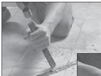
In some situations a small channel may have to be made in the floor to accommodate the tubing. If so, cut a channel from the thermostat position approximately 20-30cm across the floor.
