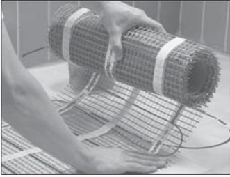
Remove the plastic outer and place the cold tail of the mat at the connection point. The Devimat™ has a self-adhesive backing, lay this to the floor and roll the mat out, if necessary the mat can be laid with the cable face down. In situations where the mat has to be turned over it can be secured using Devipins, hot glue gun (taking care not to damage the heating cable), staple gun or double sided tape.
